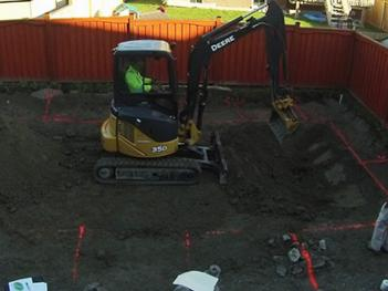
Keep the measurement points you made clear at all times. If necessary remark the measurement points during excavation. Use the grade rod and level once the excavator operator is getting close on the depths by placing the grade rod into the hole immediately adjacent to one of the measuring points that you made.
