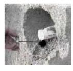
This lens assembly should glue directly on 1 ½" PVC pipe. DO NOT GLUE A REDUCER BUSHING DIRECTLY INTO THE LENS HOUSING! If you want to reduce to 1" PVC pipe, do so with a reducer after a few inches of 1 ½" PVC pipe. This is to allow room for the lens assembly to seat into the body of the lens housing. The LNS-2G & LNS-2GB housings must be installed 12" to 14" down from top of wall.
